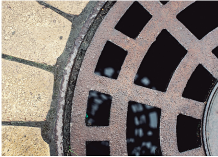
Stormwater Runoff Drains
